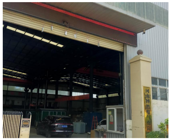
项目南侧搏然电气
